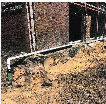
Temp sanitary ejector line installed to allow excavation to continue for proposed new elevator pit.
