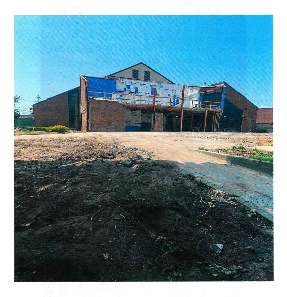
Building exterior demolition completed. Partition wall separating the main core library to have Tyvek, waterproof and liquid membrane for sealing the remaining perimeter.
