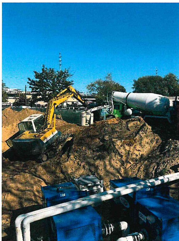
Stalco, Subcontractor York pouring the concrete for the required underpinning for the new elevator pit.
